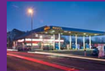
Spar Filling Station Ahoghill 2006
